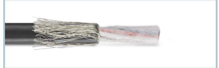
Fit the shield sleeve on the cable
